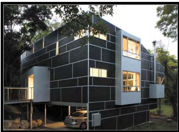
Decorative H3 treated plywood cladding (Courtesy CHH WoodProducts Australia)
