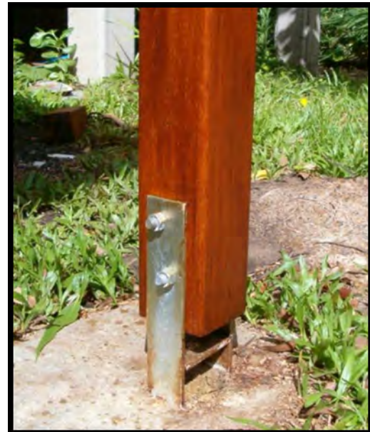
Naturally durable hardwood Glulam post isolated from ground
