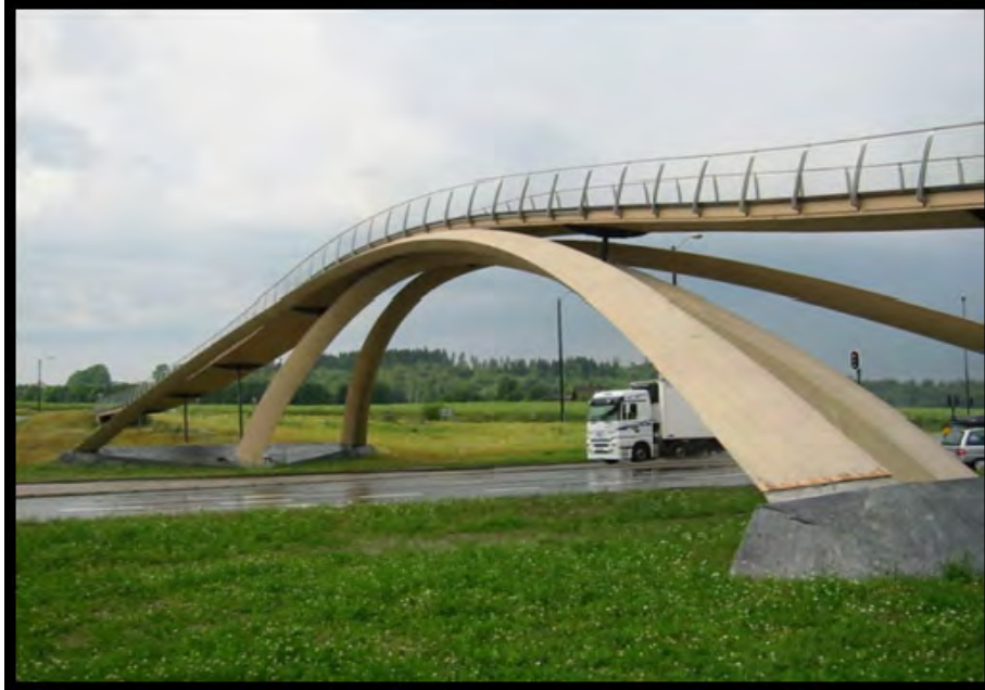
Treated Glulam pedestrian bridge, Ås, Norway (Courtesy Timber Queensland)
