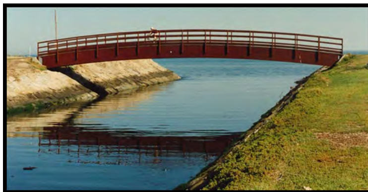
Treated Glulam pedestrian bridge in full weather exposure (Elwood Canal, Melbourne).
