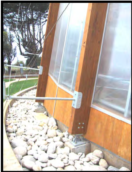
Treated Glulam and plywood structure isolated from ground (Courtesy Harry Greaves)
