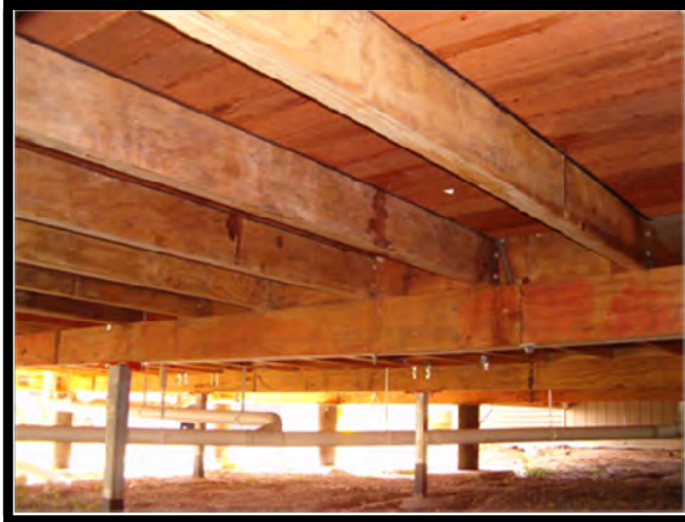
Damp proof course strip above H3 treated LVL deck joists to isolate from decking and weather (Maryborough)
