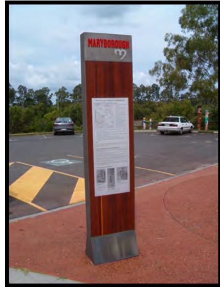
Natural durability class 2 hardwood Glulam sign post. (Courtesy Stephen Bolden)
