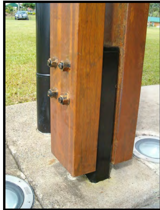
Durable hardwood Glulam column finished with semi-transparent exterior timber stain.
