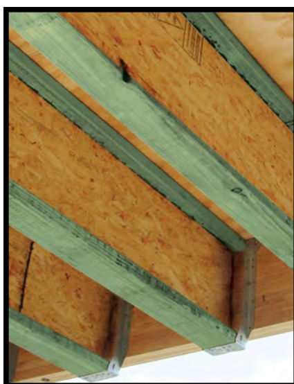
H2 treated I-beam with finger jointed flanges & OSB webs (Courtesy Hyne)
