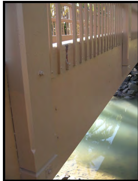
Durable hardwood Glulam bridge finished with exterior paint (Airley Beach, Qld).
