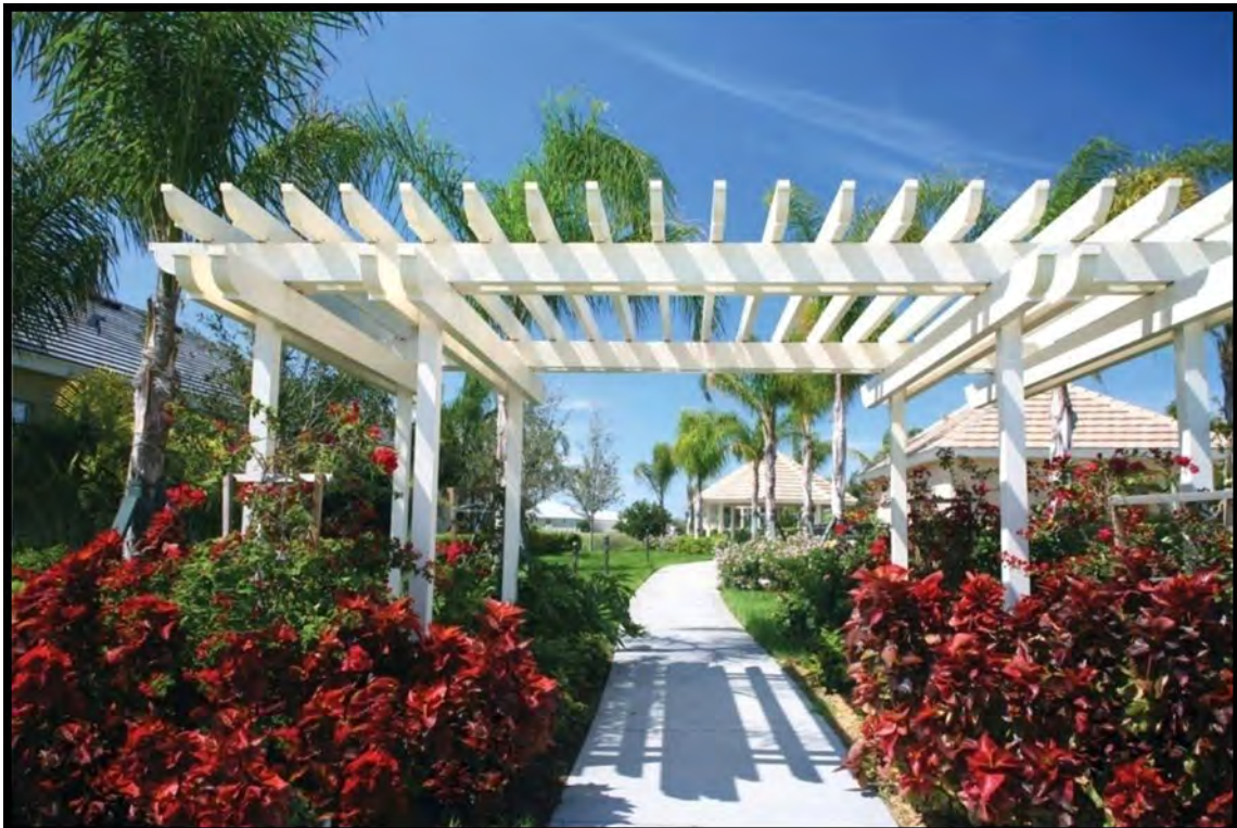
Pergola constructed from pine Glulam, H3 treated, primed and painted for full exposure to weather. (Courtesy Hyne)
