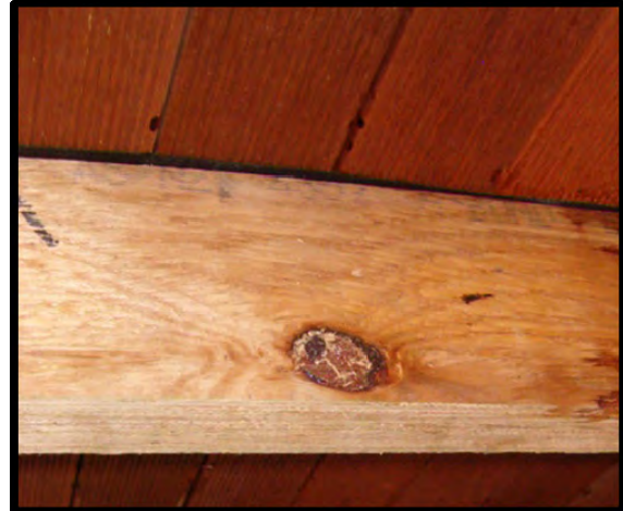
Damp proof course strip above H3 treated LVL deck joists to isolate from decking and weather (Maryborough)
